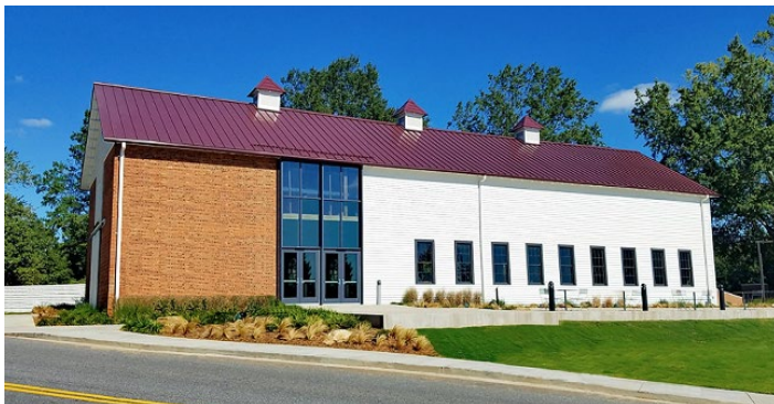
The renovated Barnes Center. Photo courtesy of MMSA Structural Engineers
