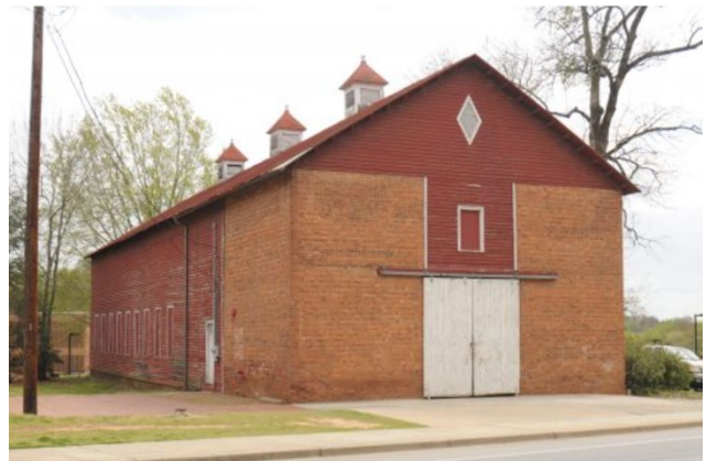
The Sheep Barn before renovations. N.d. Photo courtesy of Clemson Blogs .
