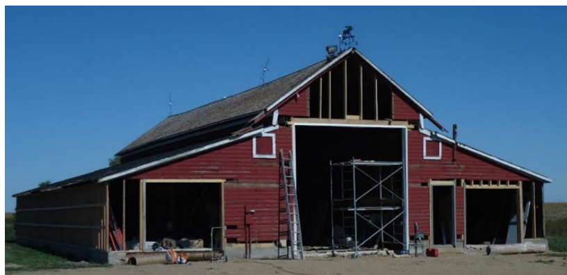
The Levee Farm Barn Under Construction. Photo courtesy of Kristen Catherwood .
