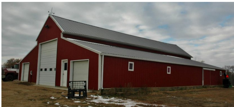
The Levee Farm Barn circa 2013. Photo courtesy of Kristen Catherwood .
