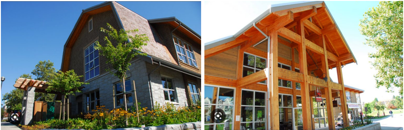
The Old Barn Community Centre. Photos courtesy of UBC Properties Trust
