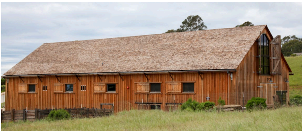
The reconstructed Hay Barn. Photo courtesy of UC Santa Cruz Center for Agroecology .
